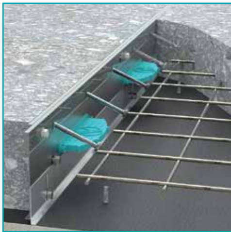
» RIGHT AFTER POURING CONCRETE
