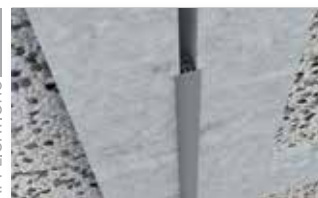
50 mm gap for stainless steel corner
